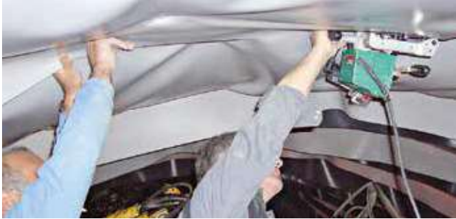
Comet operating in the tunnel ...
