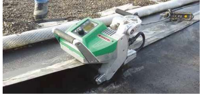
The GEOSTAR welds nearly 240 m without difficulty in a single pass during a field test (South Africa)..
